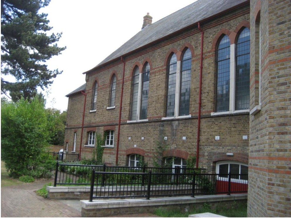
Figure b.1.4 Left-hand side of the Normansfield Theatre.
