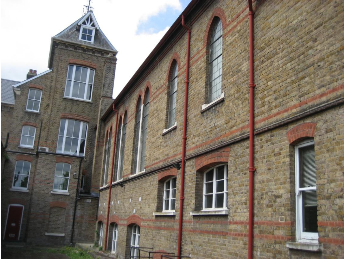
Figure b.1.3.1 Rear of the Normansfield Theatre.
