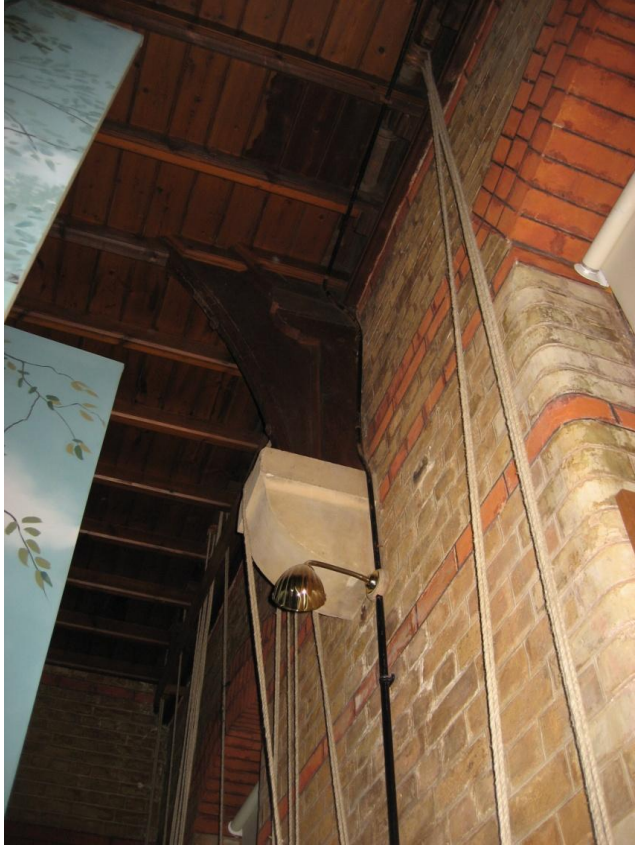
Figure b.1.12 The original rope rigging system used at the Normasfield Theatre.
