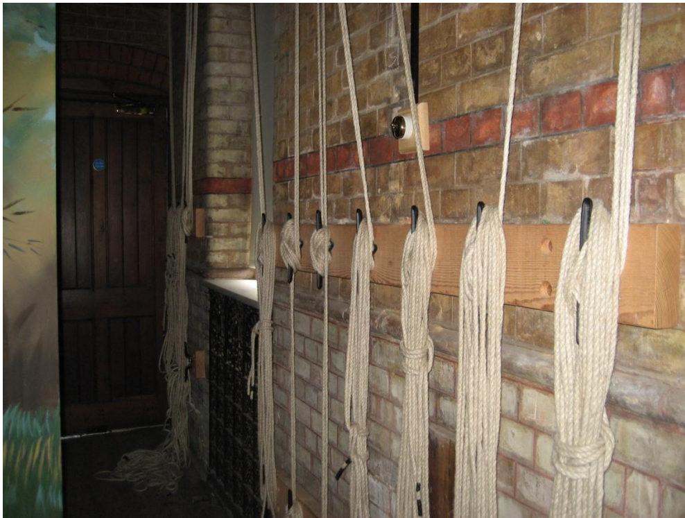
Figure b.1.13 The original rope rigging system used at the Normasfield Theatre.
