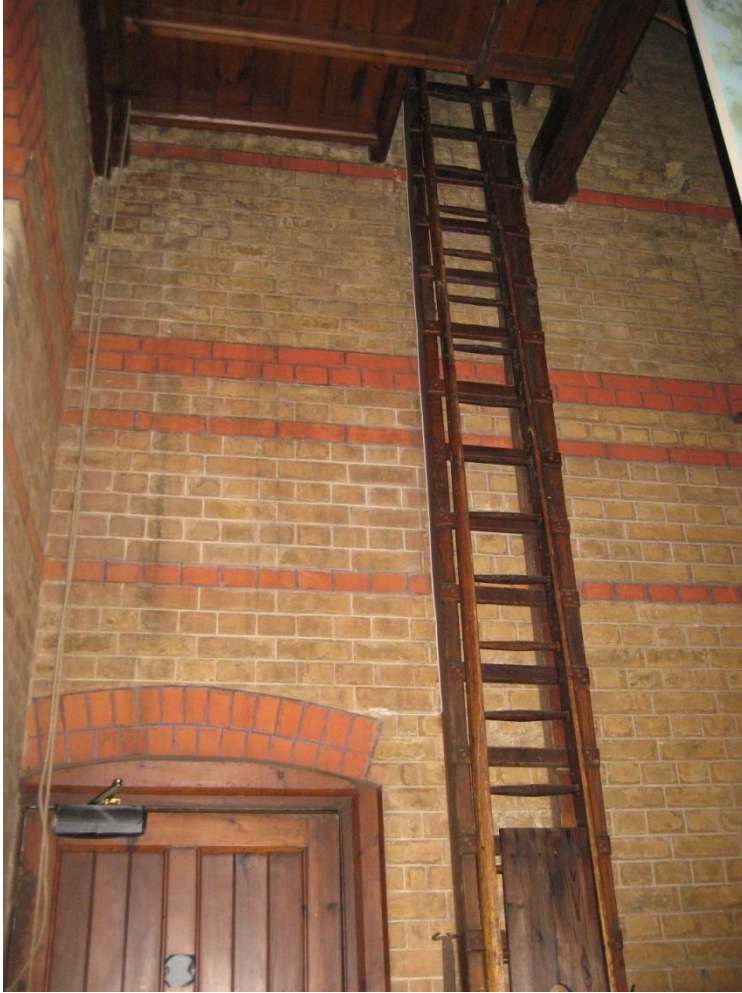
Figure b.1.15 This is a ladder used to access the rigging of the Normasfield Theatre.
