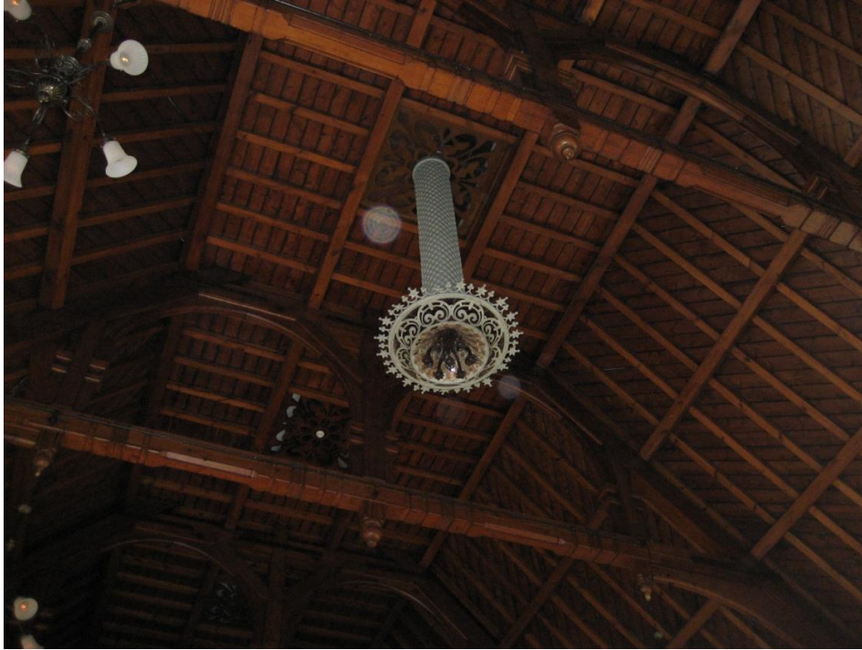
Figure b.1.7 Original gas lighting system for the seating banks.
