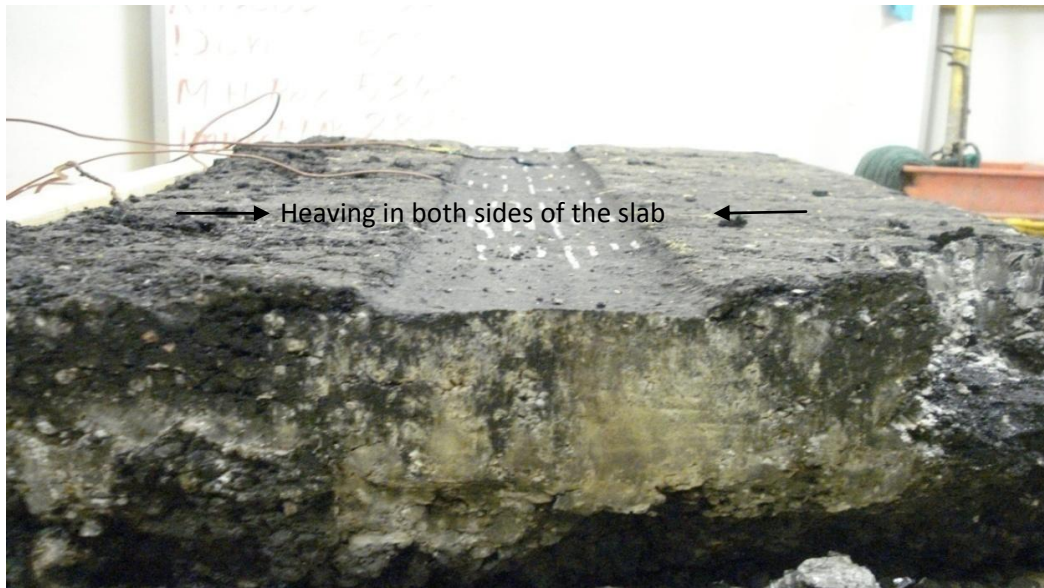
Figure 34: Rutting Inside Wheel Path
