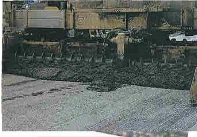
Figure 8: Ultra Thin White Topping
