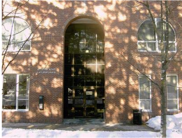
Figure 10 - Entrance to Atwater Kent
