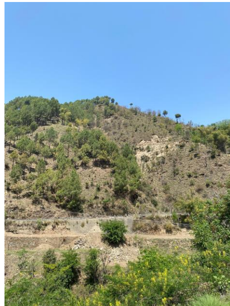
Figure 12: Dry mountain slopes from long periods of lacking rain and snowmelt tend to lead to more landslide activity (Photo credit: Fox).
