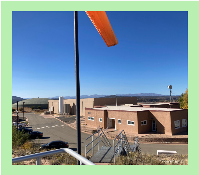
Buckman Direct Diversion Water Treatment Plant
