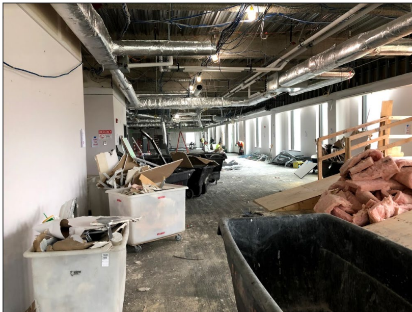
Figure 18: Site Walk Photo – Demolition
