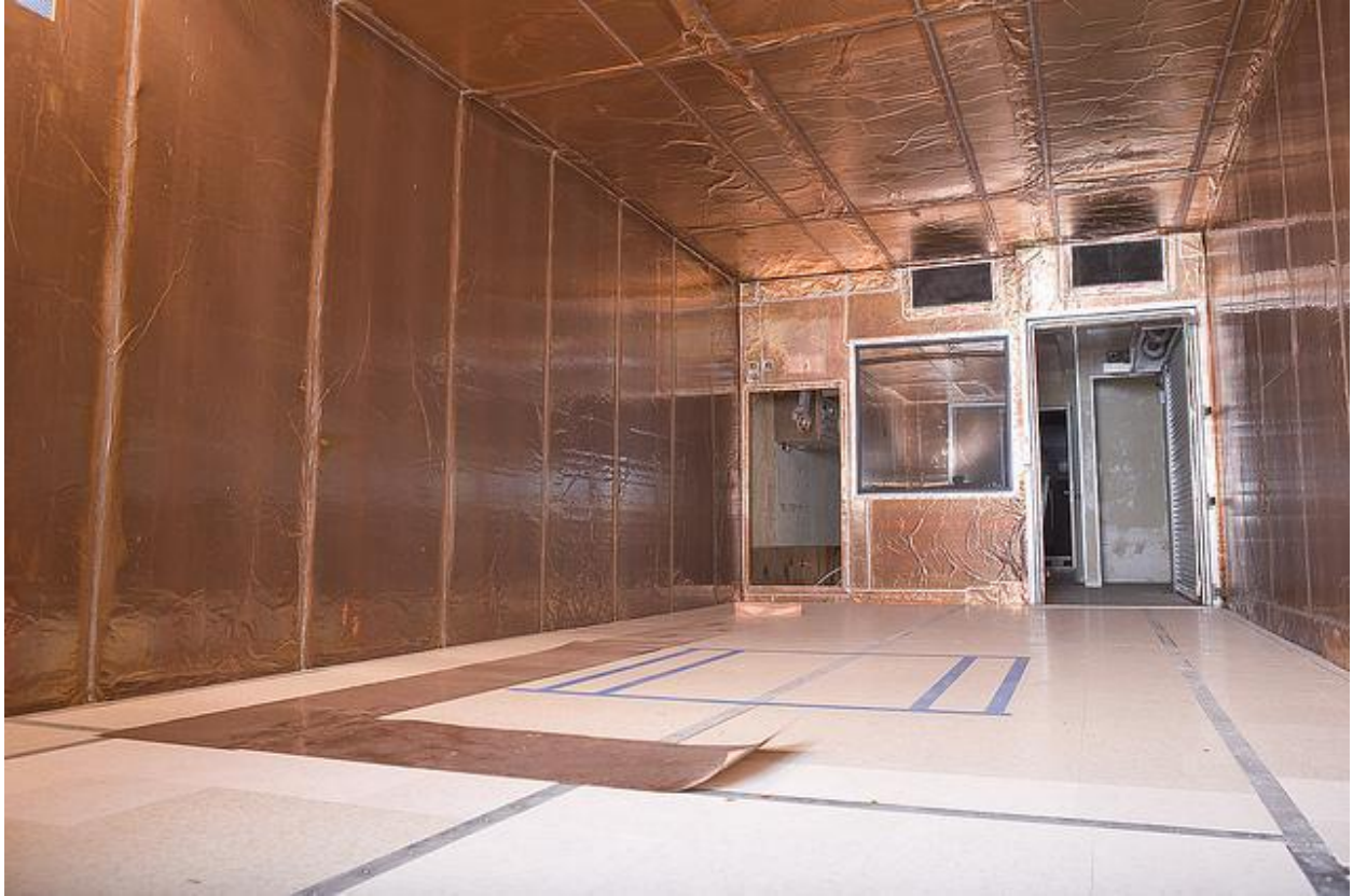
Figure 3: Copper RF shielding in a planned MRI room
