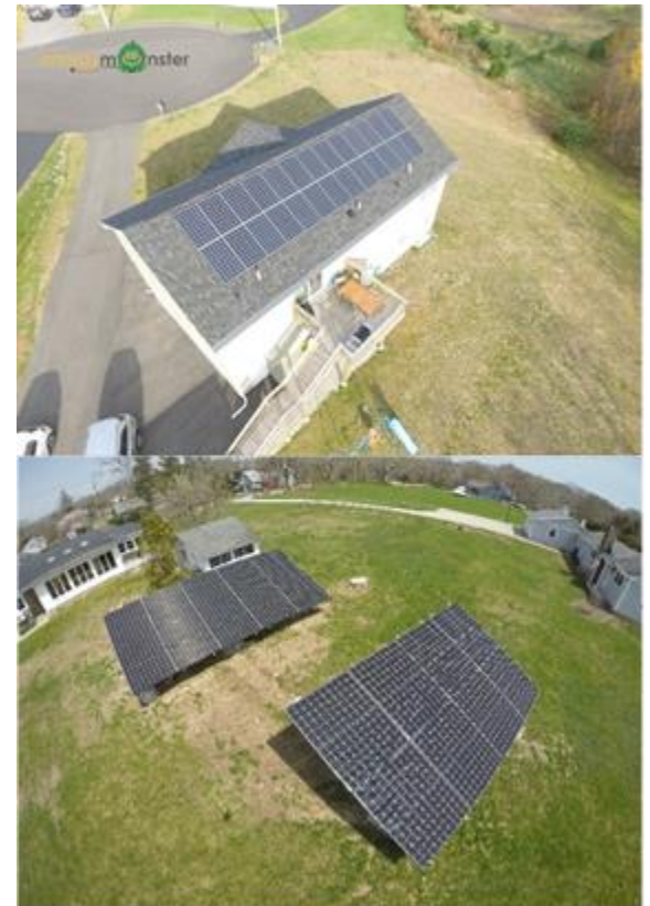
Figure 14: Roof mounted solar panels (top) compared to ground panels (bottom) (Gawrych, 2019)
