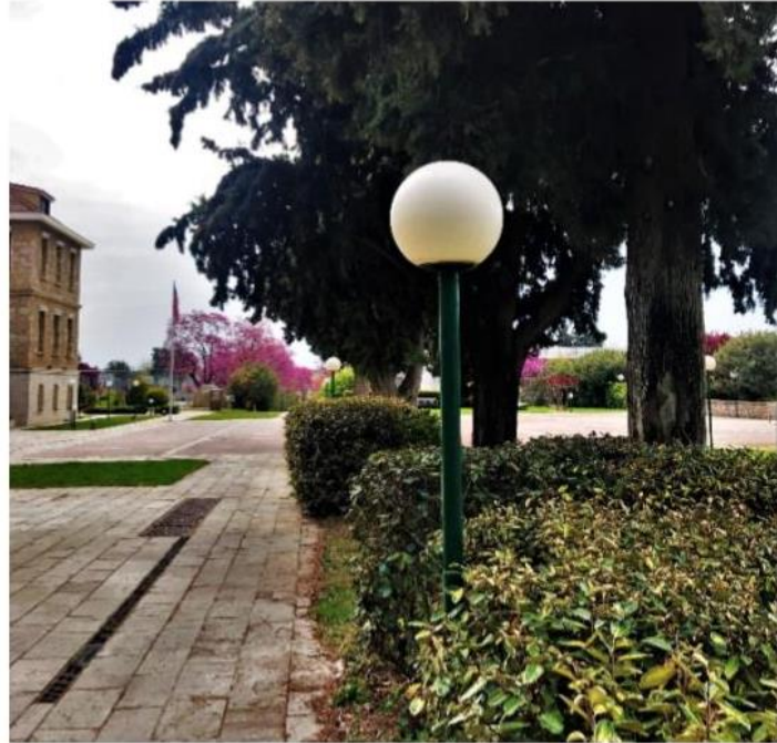
Figure 10: Example of an ineffective outdoor light that is negatively contributing to light pollution on the AFS campus
