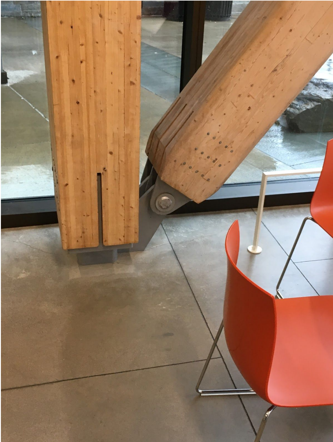
Figure D3: Angled Spline Connection
