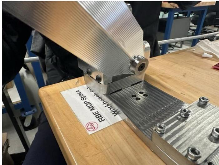
*Figure 8.8: Attaching the Ground Link to the front of the Ankle Roll Coupling via a Bottom Mount of Rotational Adjustment Piece*
