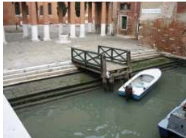
Figure 2-2: Example of a dock over-structure
