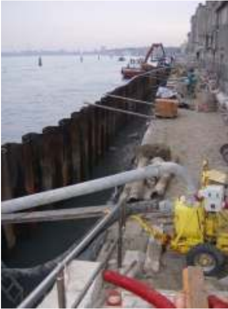
Figure 27: The vertical technique used to dredged in The Grand Canal is also used for various locations throughout the lagoon
