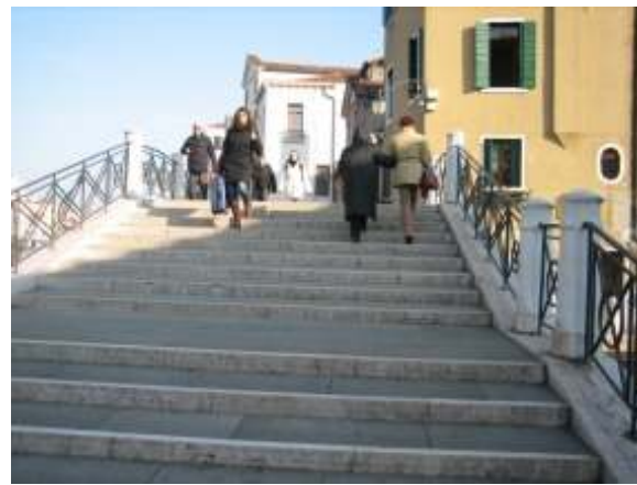
Figure 47: Head-on view of Ponte de la Croze
