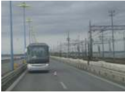
Figure 1: bus traveling across the viaduct bridge from the mainland
