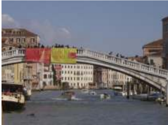
Figure 2-3: The bridges of Venice allow pedestrian and vehicular traffic to never intersect
