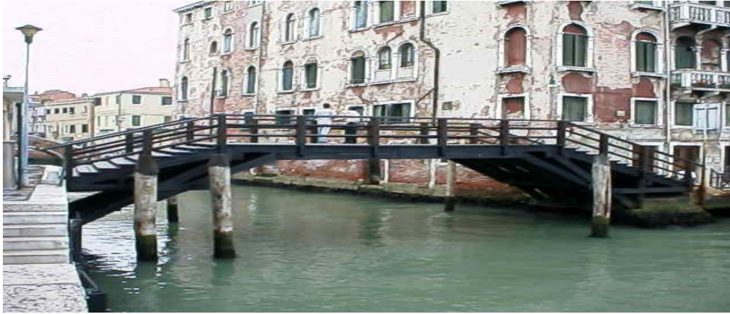
Figure 6- Ponte Molin, an example of a trapezoidale bridge
