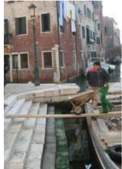
Figure 11- Temporary structure to enable workers to use a useless dock
