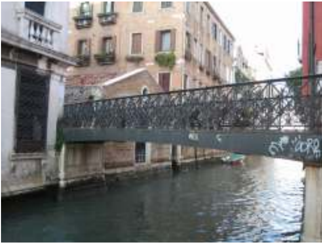
Figure 15: Side view of Ponte de la Bergama
