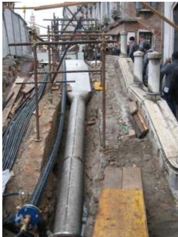
Figure 20 - A bridge under repair showing the exposed utilities
