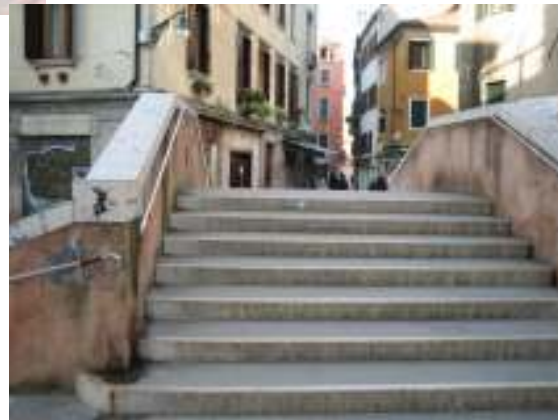
Figure 26: Head-on view of Ponte Canal
