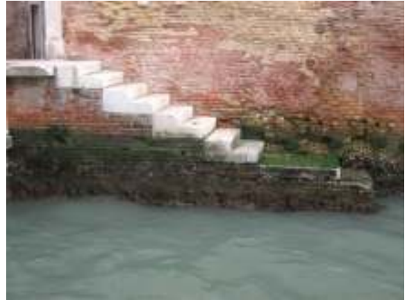
Figure 8- A versatile dock with stairs parallel to the canal
