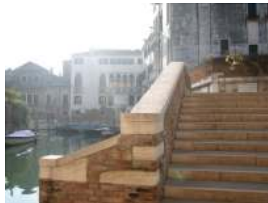
Figure 38: Head-on view of Ponte de Ca' Marcello
