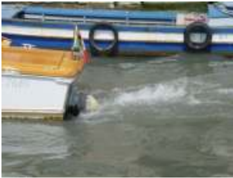
Figure 17: Wake, which is one cause of canal wall damage is shown at the rear of the boat
