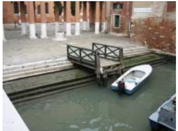
Figure 10- Wooden over-structure to help increase the usefulness of a dock
