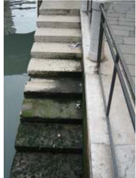
Figure 3- Dock with lower steps covered in algae
