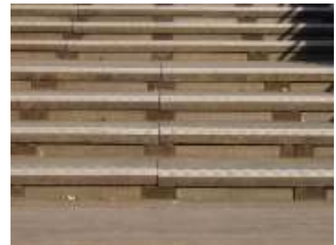
Figure 15– Metal Strips are added to wooden bridges to help those visually
