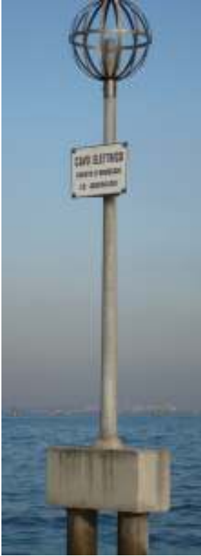
Figure 1: To install utilities within the city, many of the resources had to first be brought to the island by means of submerged pipes crossing the lagoon. These pipes are marked by poles such as the one above to indicate the potential danger for nearby boats
