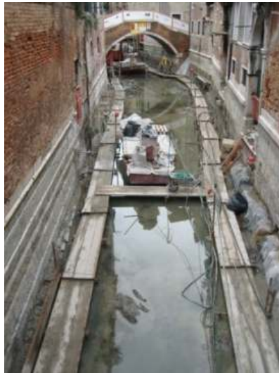
Figure 25: A canal being dredged as part of Insula's scheduled maintenance plan
