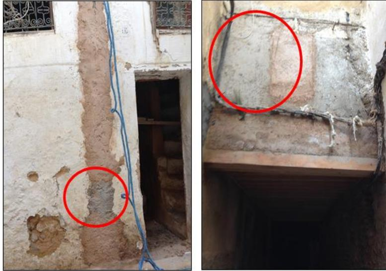
**Figure 53:** Cement mortar mixed inappropriately with traditional lime mix
