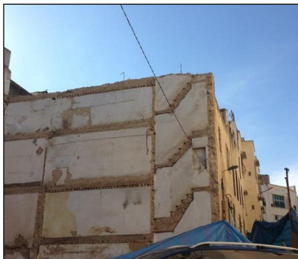
**Figure 48:** A decayed structure in the medina. The entire building has been sheared off
