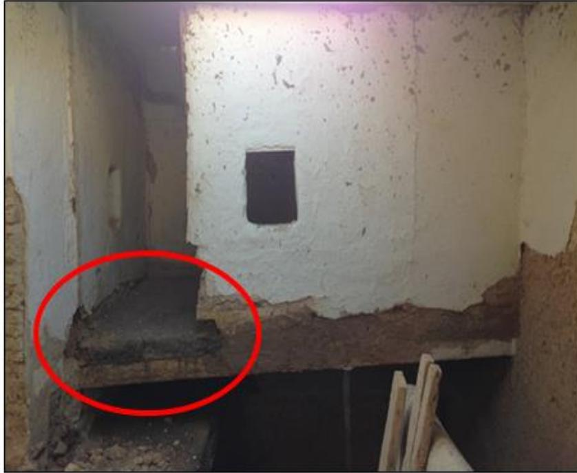
**Figure 52:** Slab using cement for flooring
