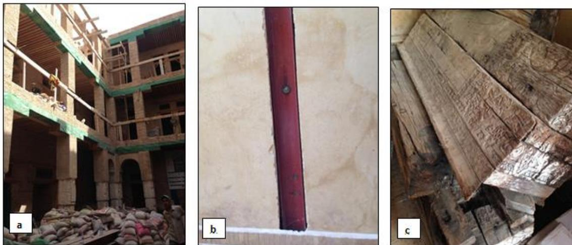
**Figure 54:** a) *Founduk* under restoration; b) C-column put in place for structural purposes; c) The original columns that will be placed in the C-column to keep original look
