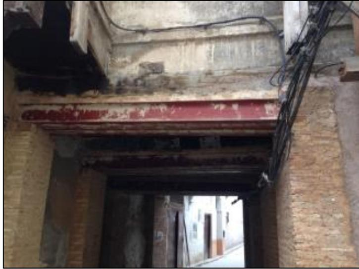
**Figure 55:** Under passage with steel beam exposed
