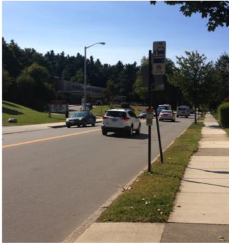
Figure 2: View of Highland Street
