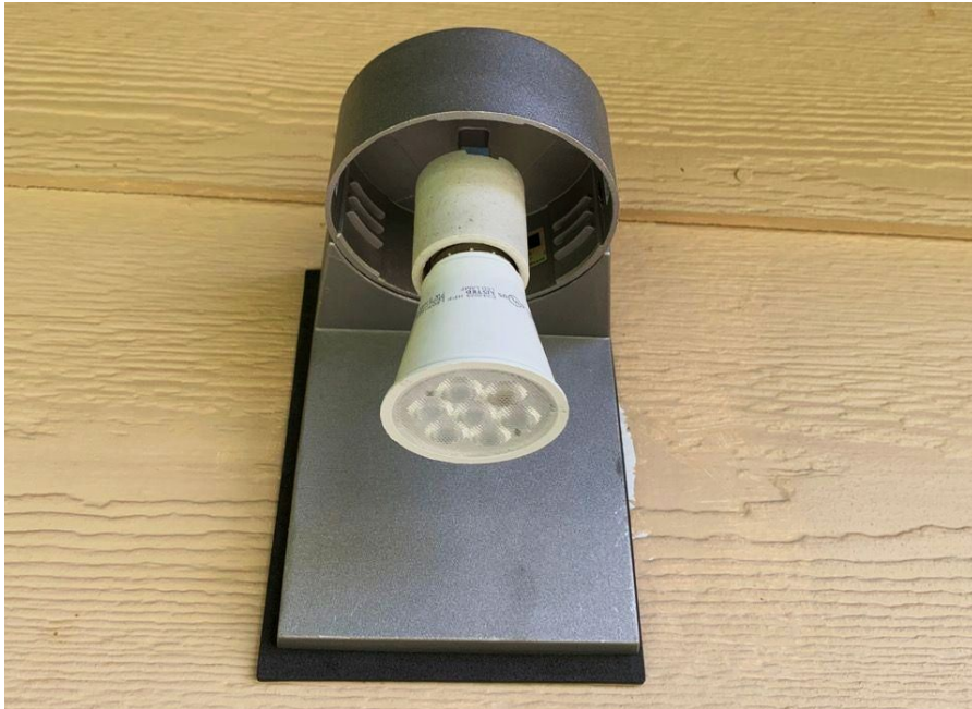
Figure 48. Dark sky compliant shielded bulb installed on a house in Headquarters. Photo by Christiana Kearns.
