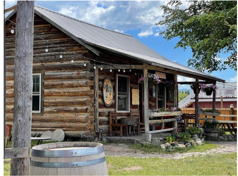
Figure 34: The Northern Lights Saloon with non-compliant string lights (R., 2021).
