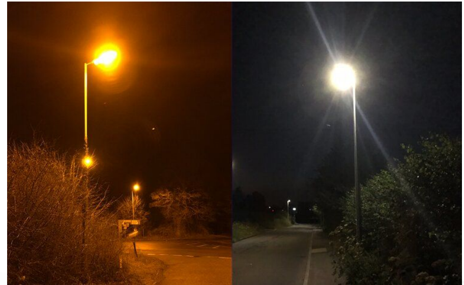
Figure 10. Comparison of warm sodium light (left) to cool LED light (right) (Boyes, 2021).
