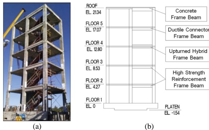
**Figure 2. Building specimen (a) skeleton; (b) elevation view (elevation in meters) [images and schematic from Chen et al. 2014].**
