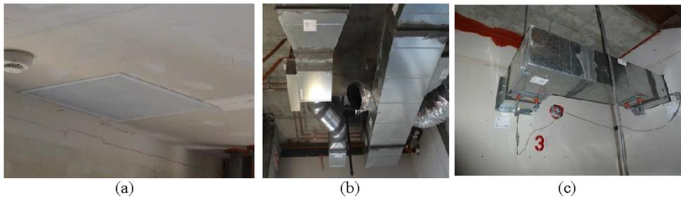
Fig. 7. (a) Diffuser in ceiling; (b) HVAC ductwork; (c) fire-stopping around duct [figure 7b from 8]
