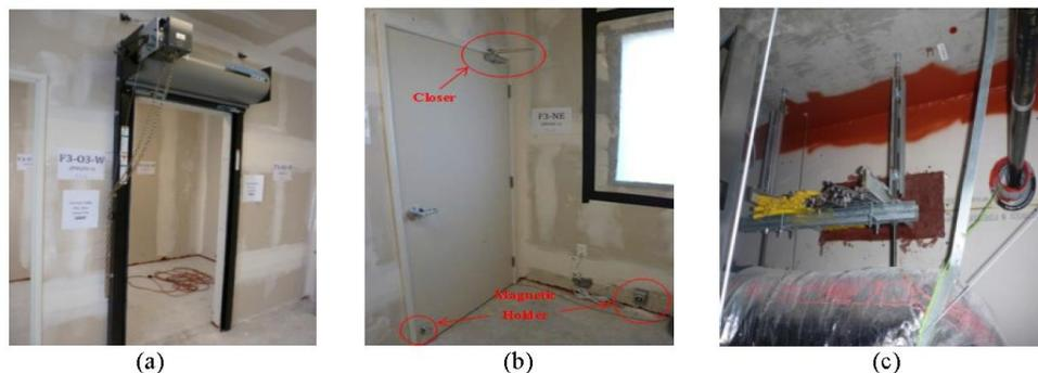
Fig. 9. Fire protection systems on Floor 3 (a) fire door; (b) door closer and holder (c) fire stop systems.
