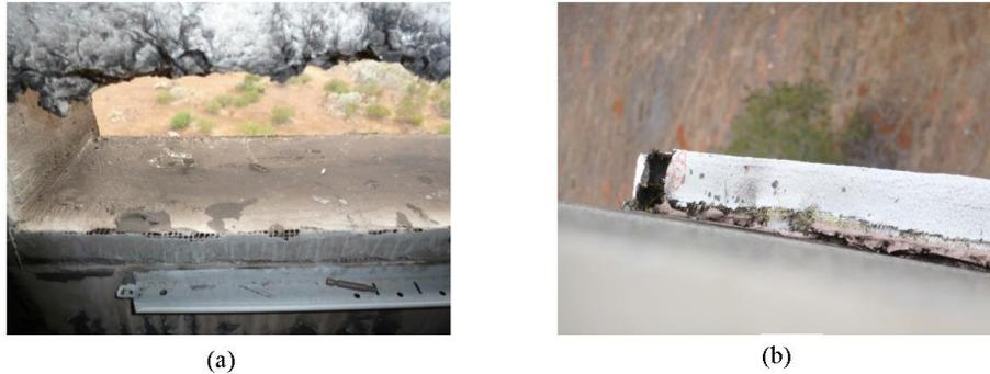
Fig. 9. Burnout of EIFS on window 4 opening (a) and smoke residue on damaged balloon framing (b)
