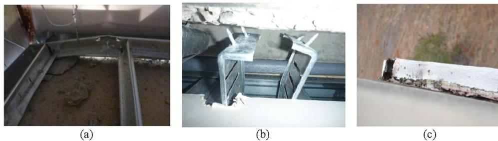
Fig. 16. Issues affecting compartment integrity (a) Gap formed at North balloon framing and ceiling joint of Floor 3; (b) detached balloon framing connection clips; (c) gaps developed at the EIFS façade.
