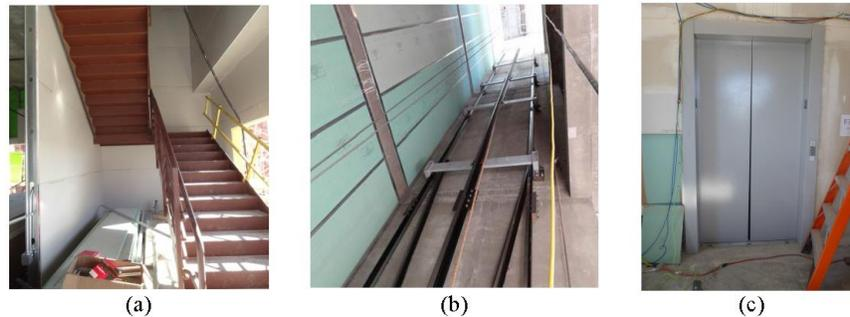
Fig. 8. Egress systems (a) stair; (b) elevator guiderails; (c) elevator door. [images 8a and 8b from 8]
