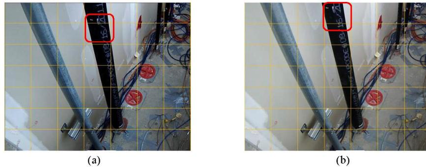
Fig. 7. Metal pipe's thermal extension: before ES (a) and during ES (b) from the 4<sup>th</sup> floor
