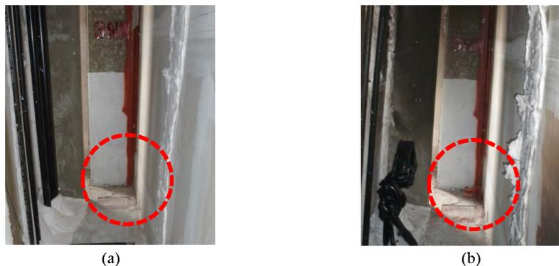
Fig. 6. Fire stop sealant before ES (a) and its fall-down after ES (b)
