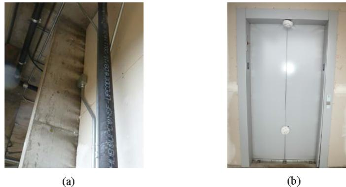
Fig. 13. Smoke spread through the gap of elevator shaft joint (a) and the gap of elevator door (b)
