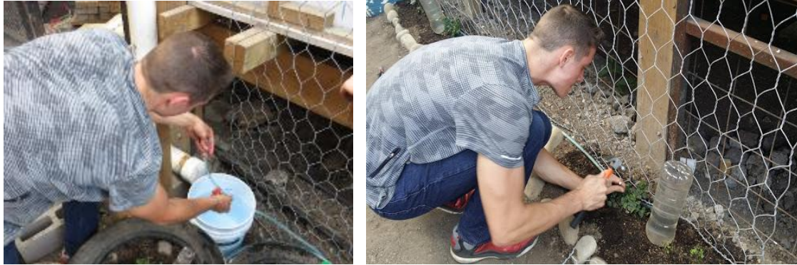
Figure 11. Installation of simple drip irrigation system for ground plants
