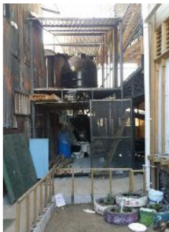
Figure 12. Shelving added above the garden area blocked sunlight from the tire gardens
