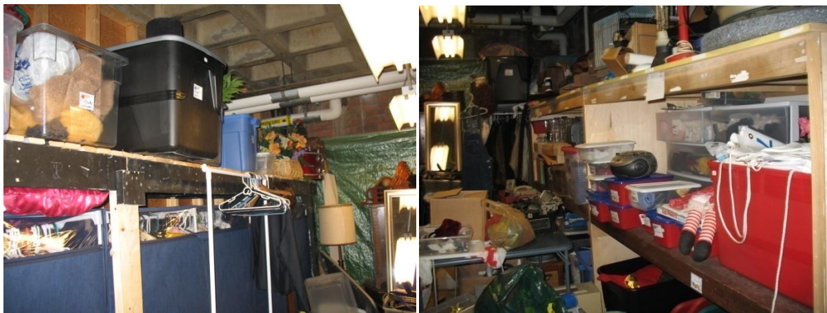
Picture 10 depicts the utter chaos of the closet before the renovation. Large containers were marked improperly and stored far out of reach. Shelves were 3 feet deep, and items in the back were rendered inaccessible.
