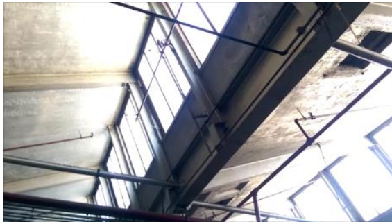
Figure 6: The Saw-tooth roof of W-3
