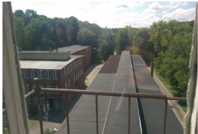
Figure 4: W-2 and the East Buildings, as seen from W-1-5.
