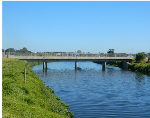
Figure 8: Valkenberg Bridge over the Black River
