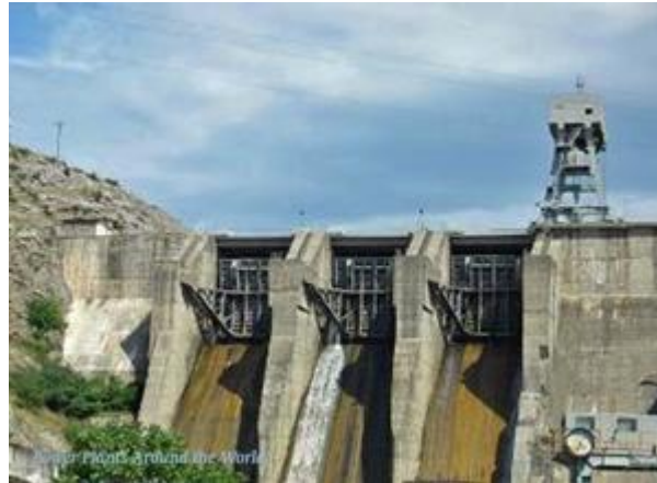
Figure 2.5: Vau i Dejës hydroelectric power plant in Albania (Platts, 2008)
