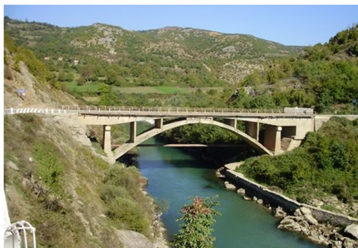
Figure 4.6: Topojani Bridge, where the float will start on day 2 (Google Earth, 2010)
