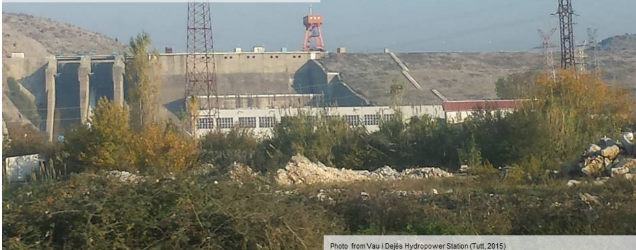
Photo from Vau i Dejës Hydropower Station (Tutt, 2015)
