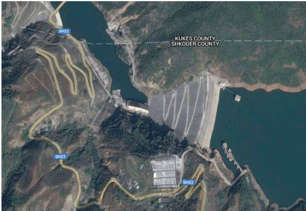
Figure 3.1: Google Earth image of the Fierza Hydropower Power Station with Lake Fierza on the right and Lake Koman on the left (Google Earth, 2015)
