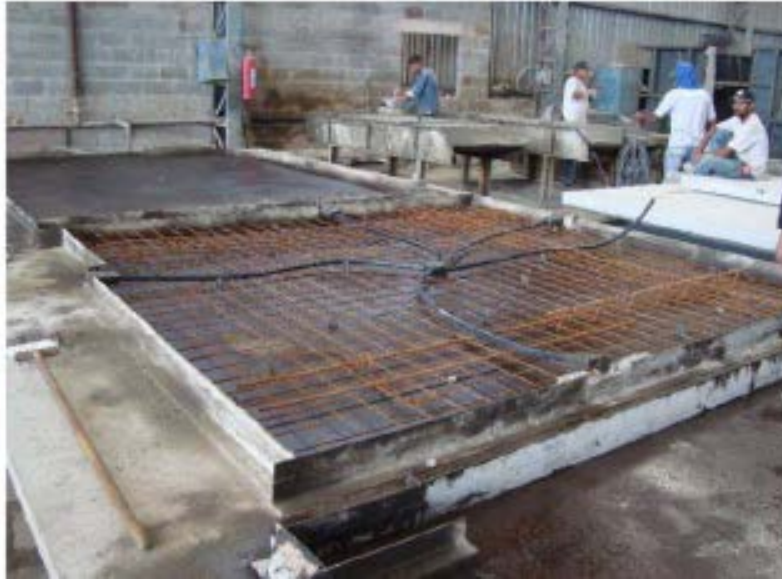
Figure 6 Pre-cast Concrete Slab Erections (Callegari, 2012)
