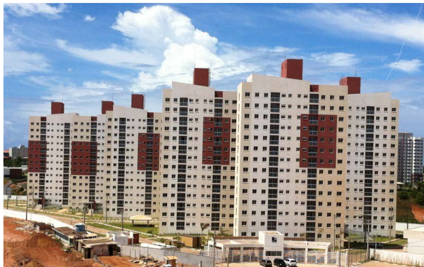
Figure 1 Structural Masonry Complex in Bahia, Brazil
