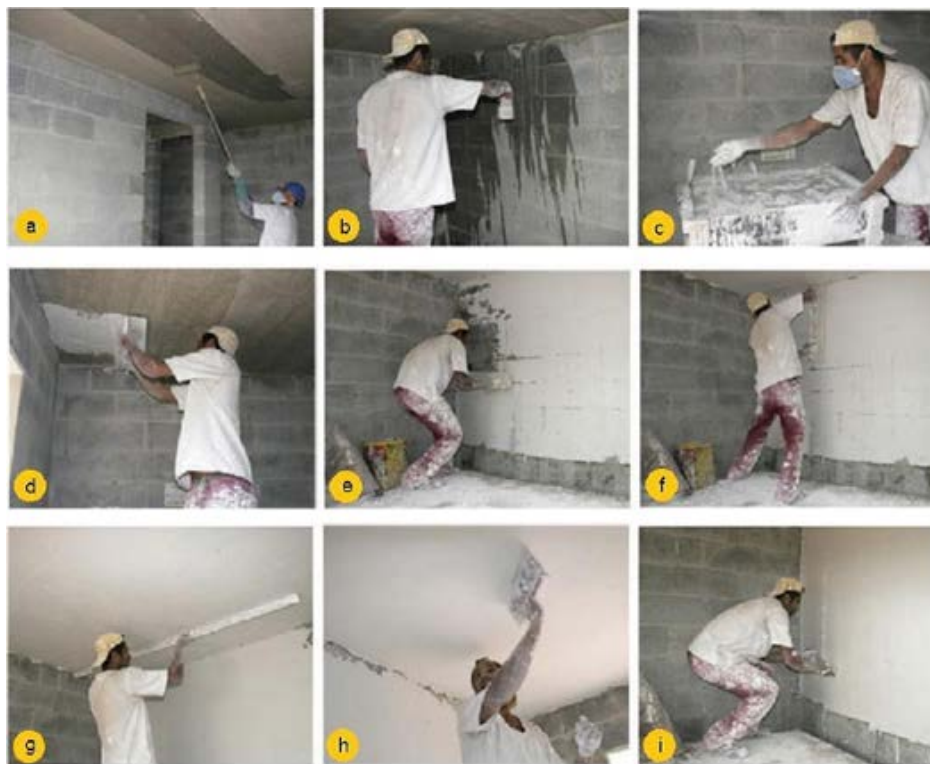
Figure 19 Process of applying finishes to interior wall (Callegari, 2012)
