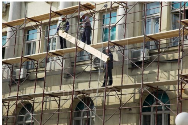
Figure 15 Typical scaffolding in the U.S. (Hunt, 2005)
