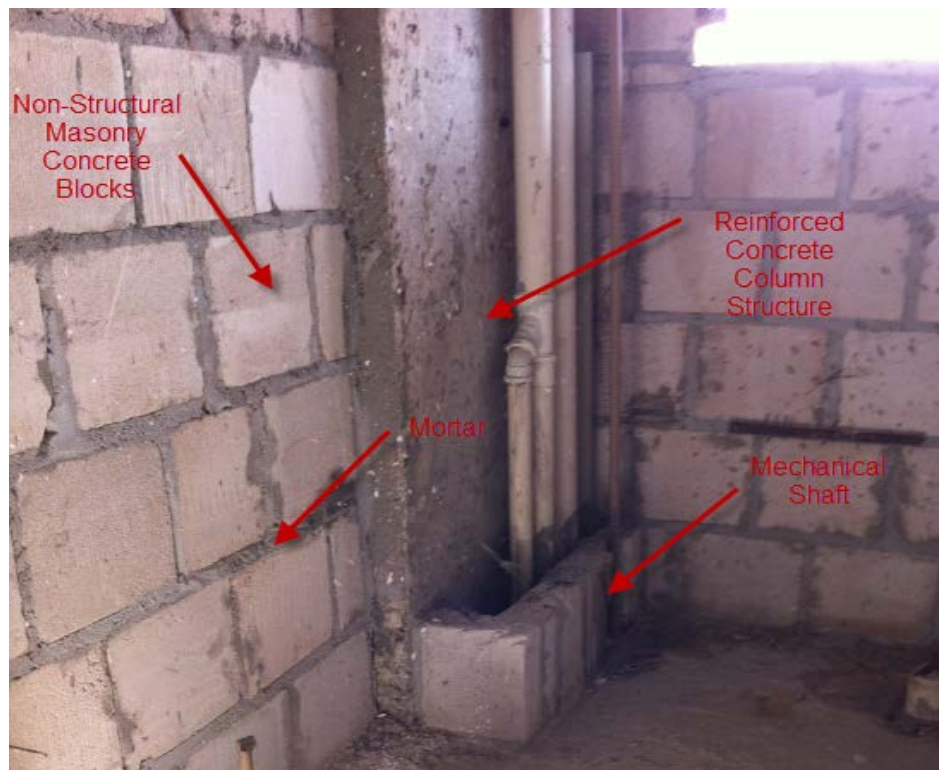
Figure 13 Corner Wall Detail (Callegari, 2012)
