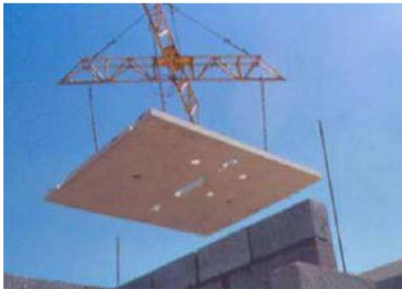
Figure 7 Pre-cast Concrete Forms (Callegari, 2012)
