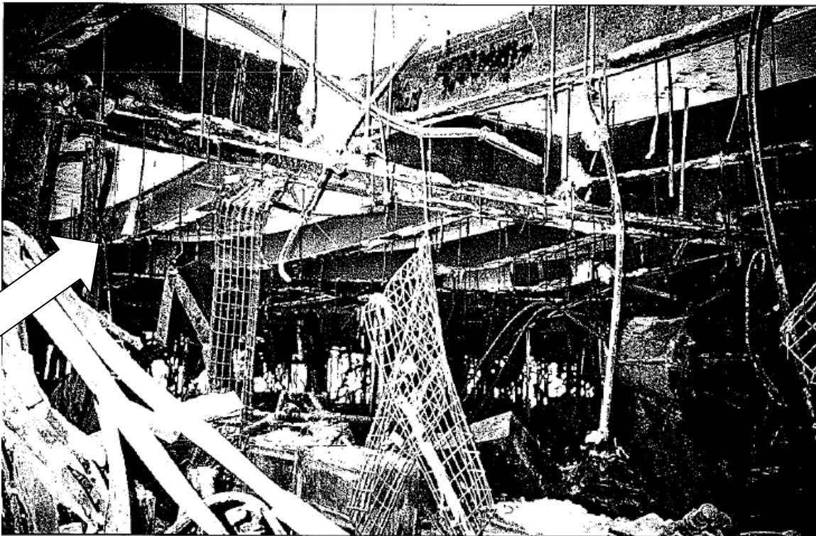
Figure 34 - Catenary Action in WTC 5
