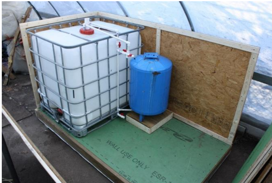
Figure 7: Inside the biodigester box, mid Phase 1
