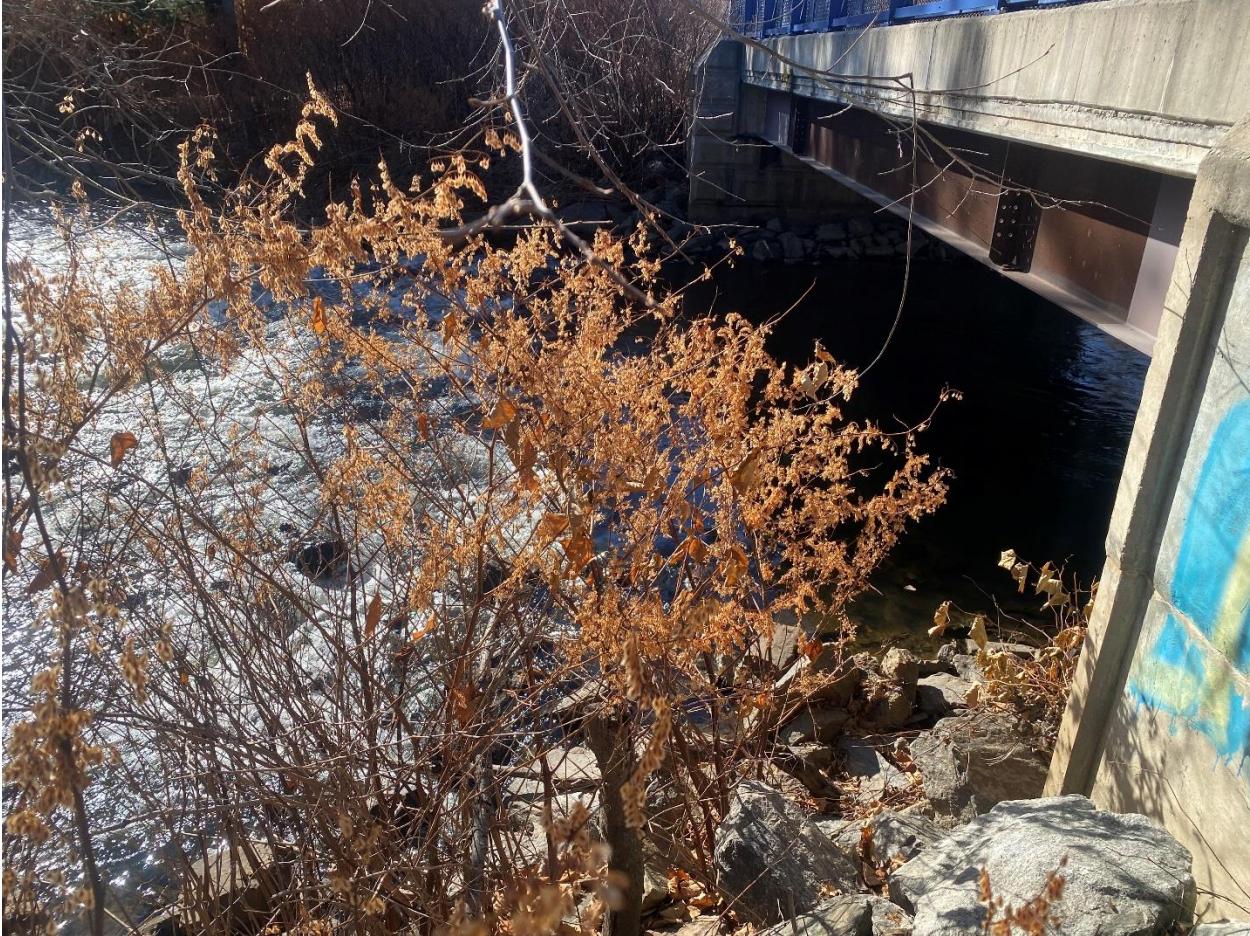
Downstream Location of Upper Blackstone (42°12'10.4"N 71°46'40.6"W)
