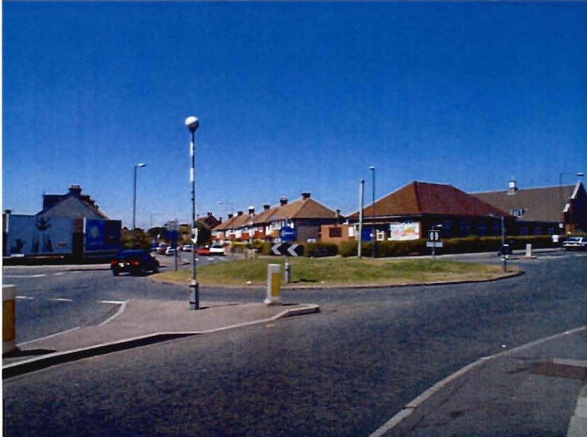
Figure 4-9 Pollards Hill Roundabout
