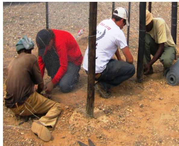
Figure 16. A finer mesh to separate compartments is attached to support poles with twisted wire
