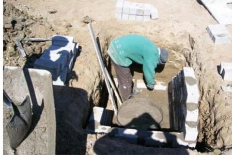
The walls of the underground tank can be built out of super bricks or any other bricks which are available. Just make sure that you keep the inside measurements shown in the construction plan. The walls must reach one brick over ground level.
