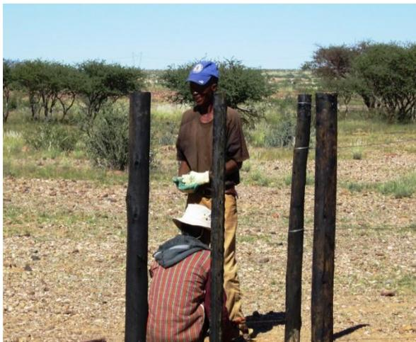
Figure 15. The first support wires are twisted around the support poles
