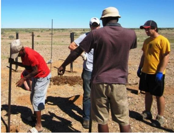
Figure 13. Hole digging using a heavy handle to separate the sand from the gravel
