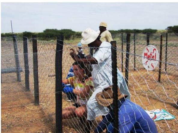
Figure 17. The penultimate layer of alley fencing is attached to the support poles
