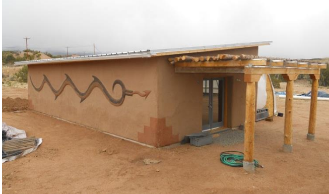
Figure 33: The Tesuque Pueblo Seed Bank, made of alternative insulating materials such as adobe, straw, and used tires.
