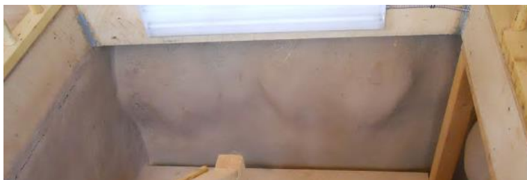
Figure 34: Bulky used tires can be seen coated in adobe mud in the basement walls of the Tesuque Pueblo Seed Bank.
