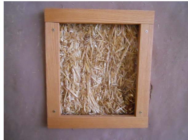
Figure 71: The 18 inch thick adobe wall of the Tesuque Pueblo Seed Bank as seen from the inside, with a square cut out showing the straw insulation on the inside of the wall.
