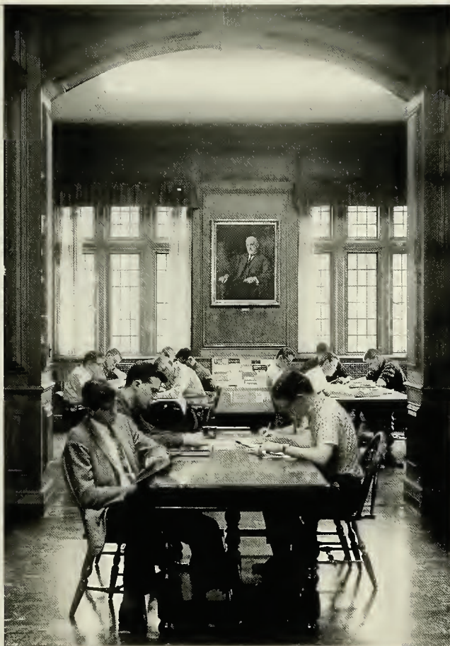
Alden Memorial, seen under construction in 1939 in the photo below, provided WPI and the Alden Trust an opportunity to honor the memory of George I. Alden, opposite. Until 1967, Alden housed the Institute's central campus library, left.
