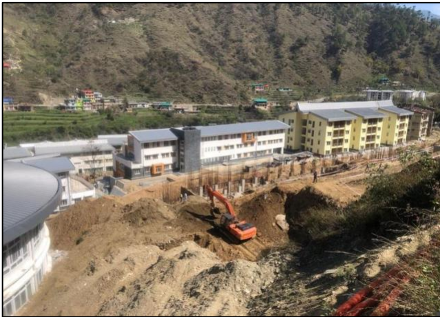
Figure 6: Cautionary zone on North Campus (Photo Courtesy: Brainard, 2019).
