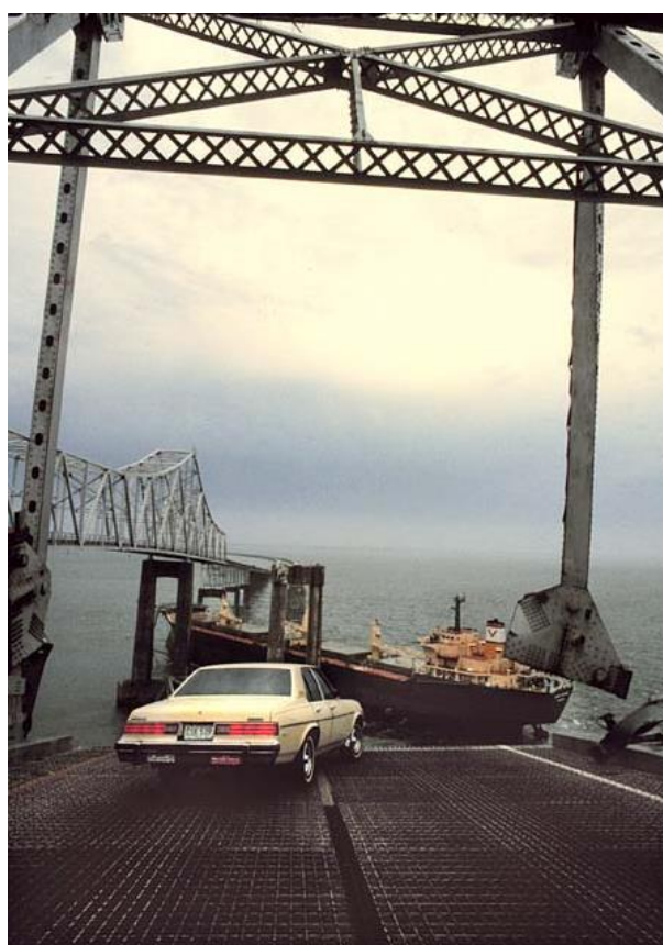
Figure 3-1. Collision-induced impact forces of waterway vessel - Sunshine Skyway Bridge in Florida
