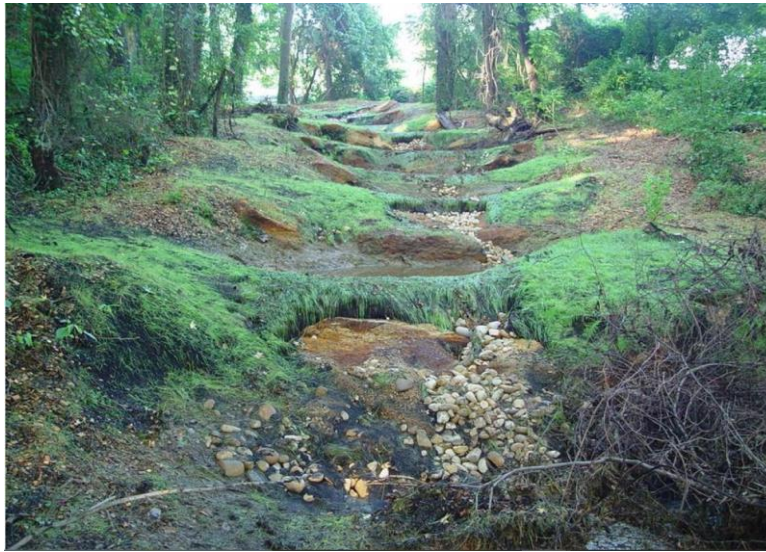
Figure 12: A Regenerative Stormwater Conveyance (RSC) under construction (Carriage Hills, 2009)
