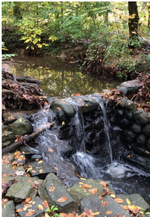
Figure 21: One of the historical dams in DOP
