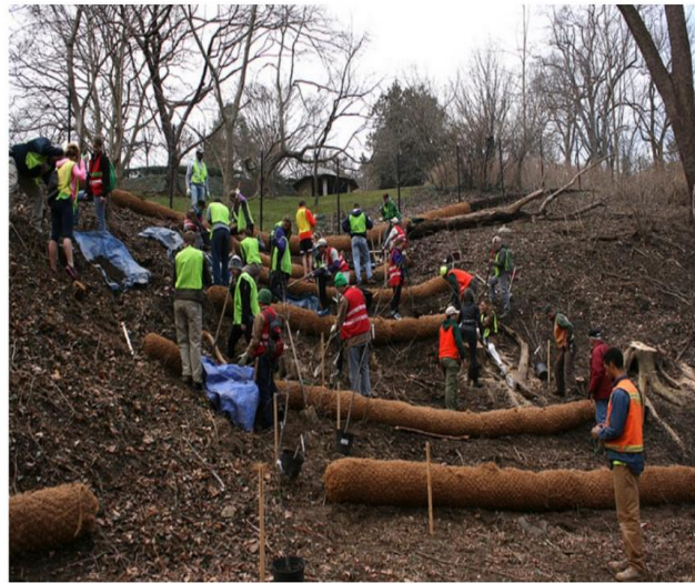
Volunteers with Casey Trees installing new trees and shrubs around the biodegradable coir logs installed earlier to decrease erosion and increase groundwater supply. Spring 2014.
