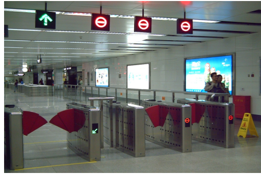
Figure 2.3: AFC on subway
