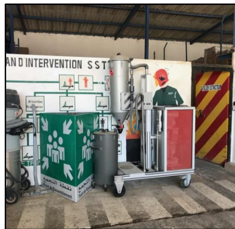
Figure 51: Fire extinguisher refill station at OCP fire department
