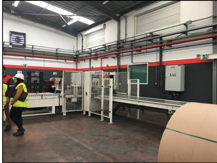
Figure 27: Exit signs in the production area leading to a corner of two walls rather than an exit
