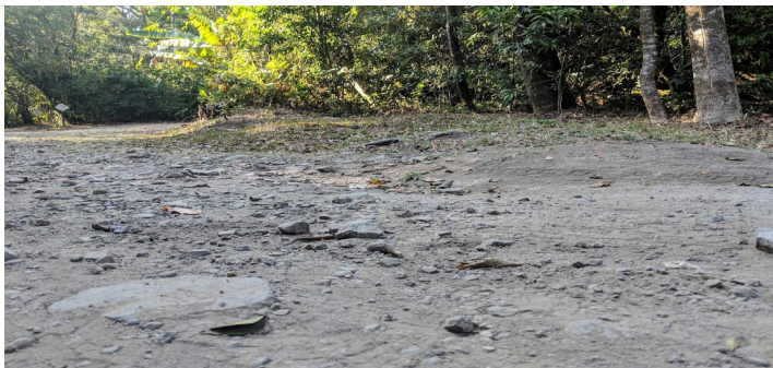
Figure 15: Current parking lot conditions
