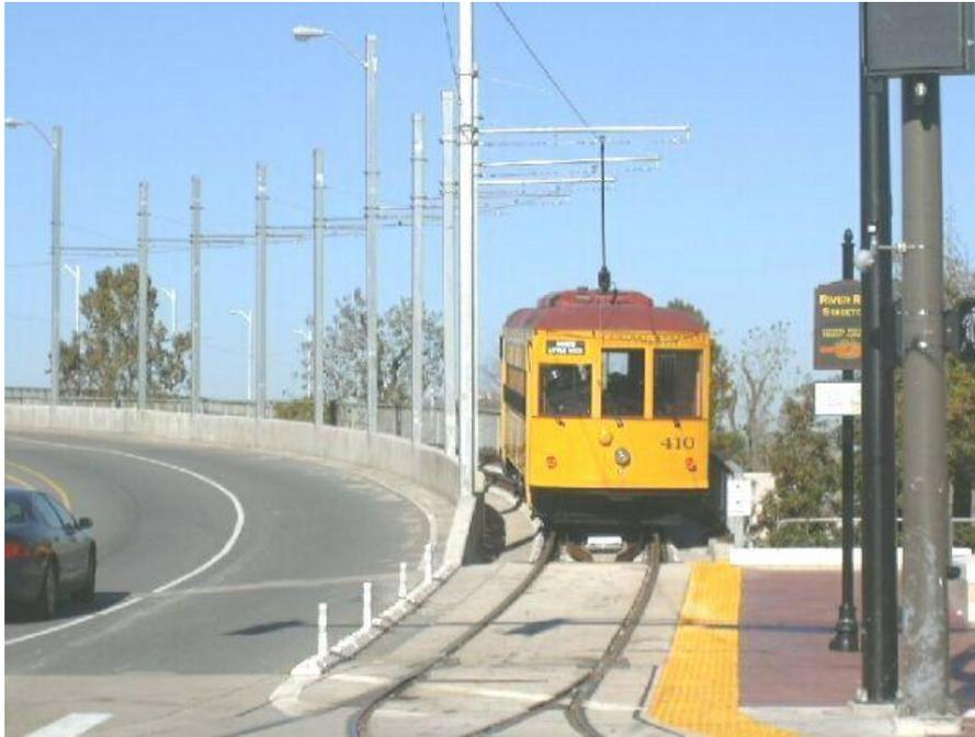
**Figure 33 - Light Rail System Appended to Existing Bridge**
