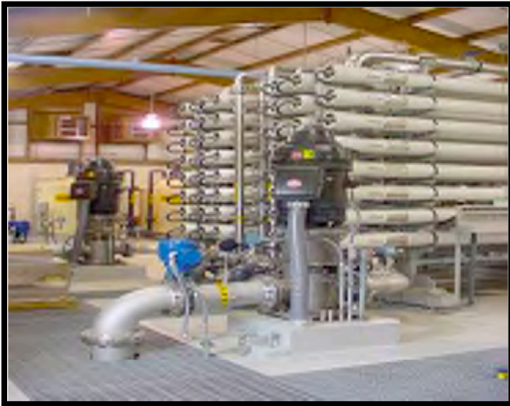
Figure 2- 1: Typical RO membrane configuration (Rojas et al., 2006)
