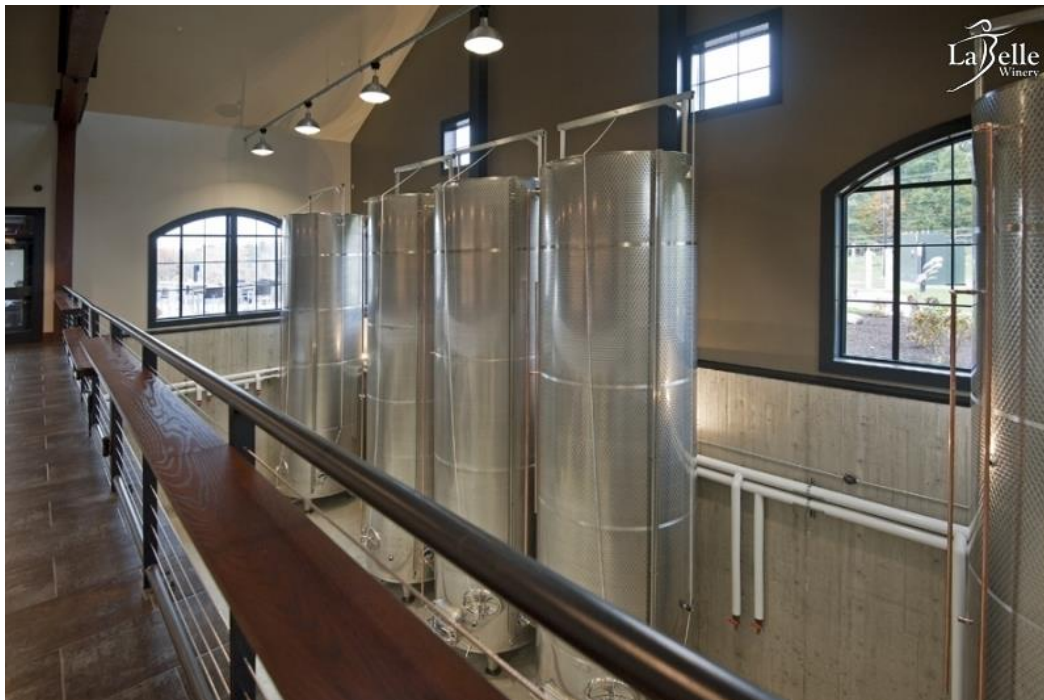
Figure 4: Five Stainless Steel Fermentation Tanks at LaBelle Winery (LaBelle)
