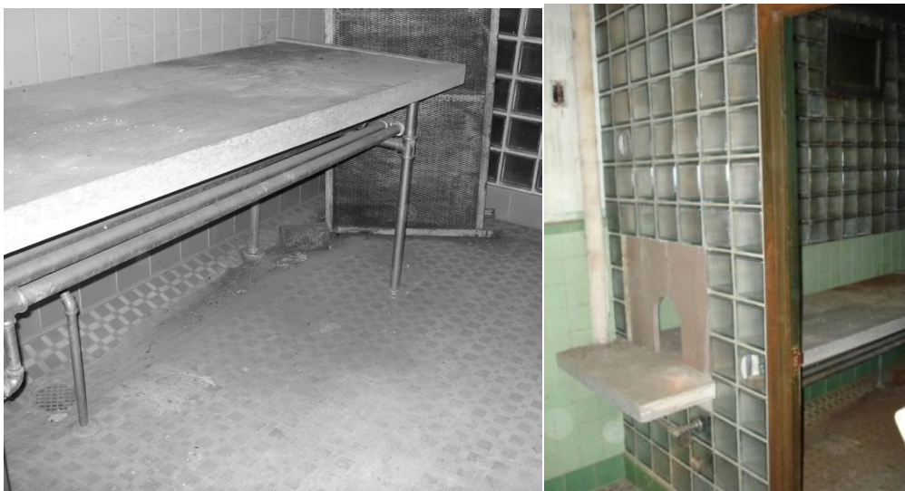
Figure 3: Interior and Exterior of Vapor bath in basement of Violent Ward of Grafton State Hospital taken in 2008
