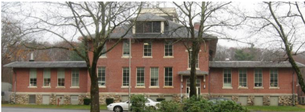
Figure 16: West face of Building 19 in fall 2008 (Tufts Era)
