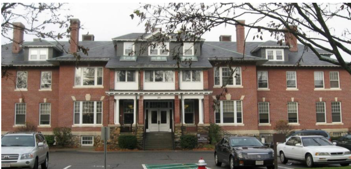
Figure 8: Administration Building in 2009 (Tufts Era)
