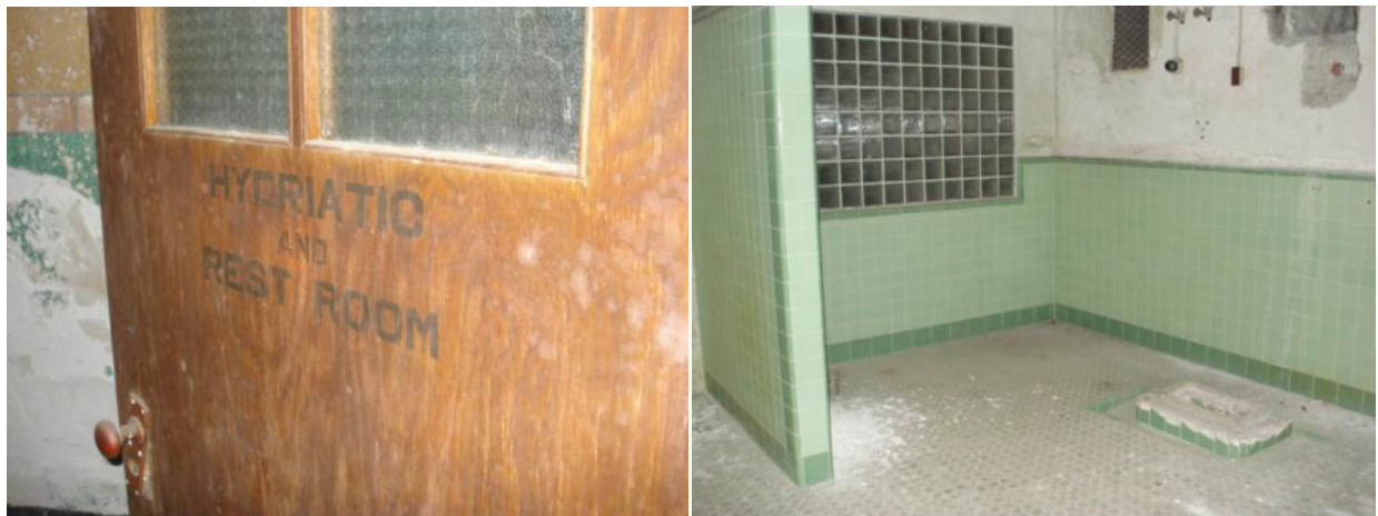
Figure 1. The Hydriatic and Rest Room at Grafton State Hospital
