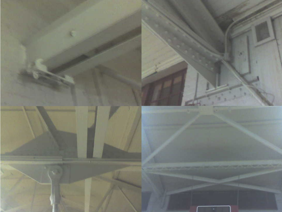
Truss System of Alumni Gymnasium Roof
