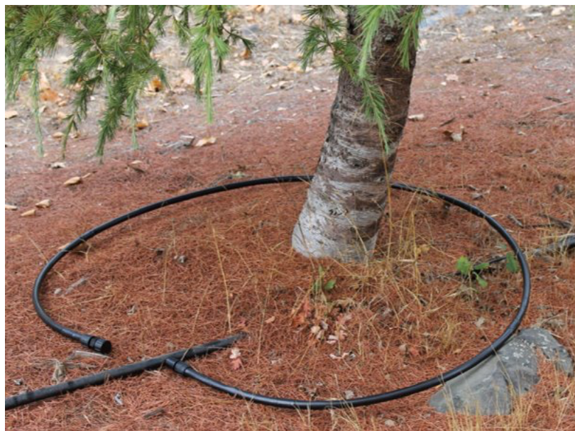
Figure 4.1 – Drip Irrigation System.
