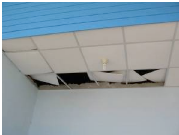
Figure 12: Displaced Ceiling Tiles in Chum Chon Tap-Parat
