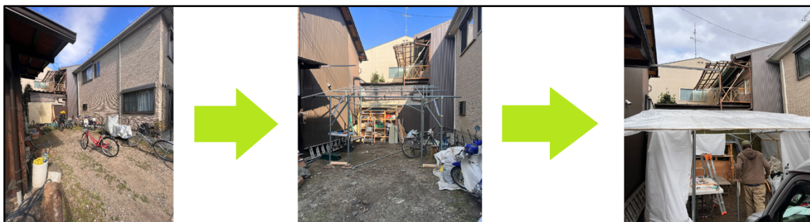
Figure 11: Image showing the construction progression of the classroom
