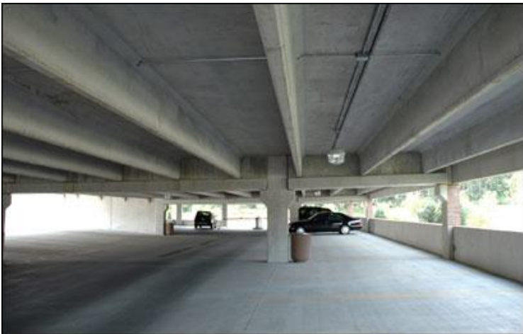
Figure 20: Double-tee Floor System [28]
