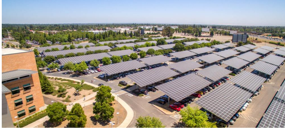
Figure 1 - A Typical Solar Canopy System (Baja Carports, 2018)
