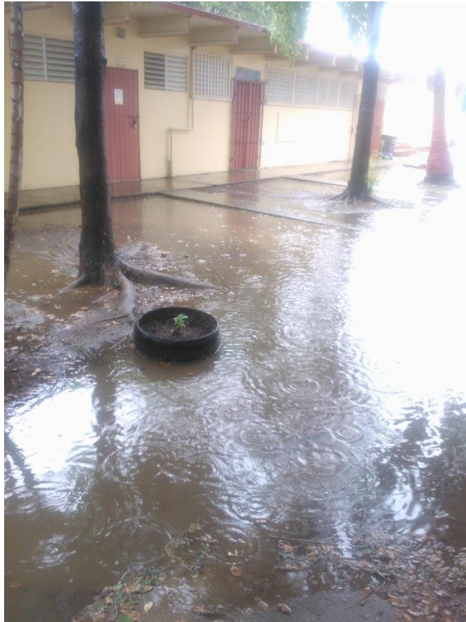
Figure 3. Flooding of School Grounds
