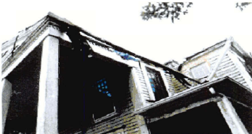
Figure 4.2(b): “Exterior Damage”
