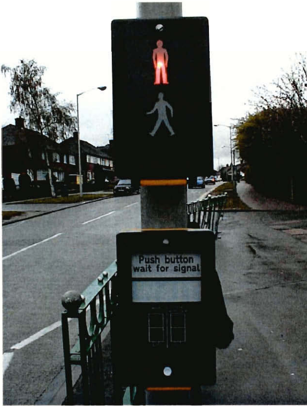
Figure 2.4: Signal for puffin crossing; notice that the ‘red and green man’ signals are above the ‘wait’ box, rather than across the street as they would be in a pelican crossing.
