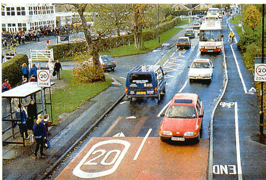
Figure 4.1: A road in front of Huntington school in York. Notice the coloured asphalt, speed hump, bus shelter and stop, bike lane, and 20 mph speed limit painted on the asphalt.
