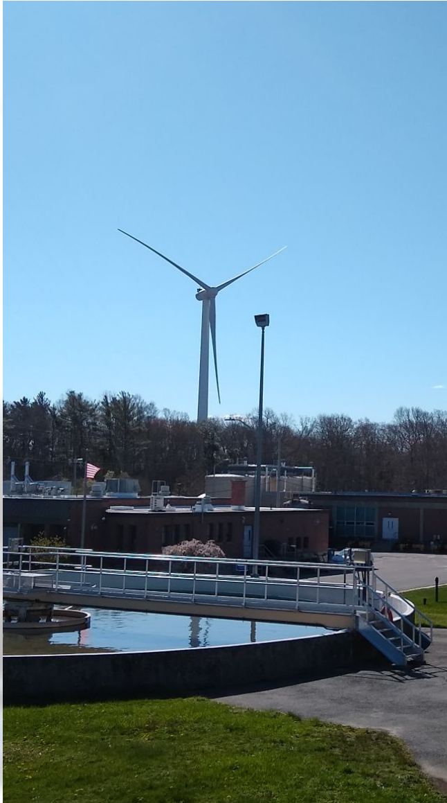
This image was taken with permission at the Fairhaven Water Pollution Control Facility at Fairhaven, MA
