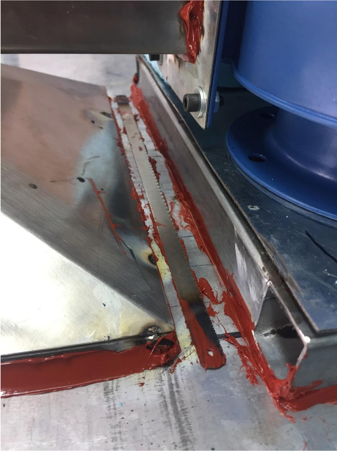
Figure 39: Some Extra Holes Sealed with the Silicone
