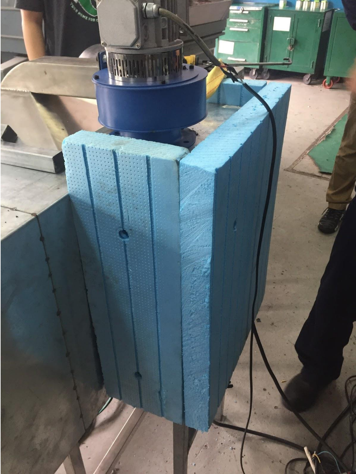
Figure 32: All Three Sides Insulated
