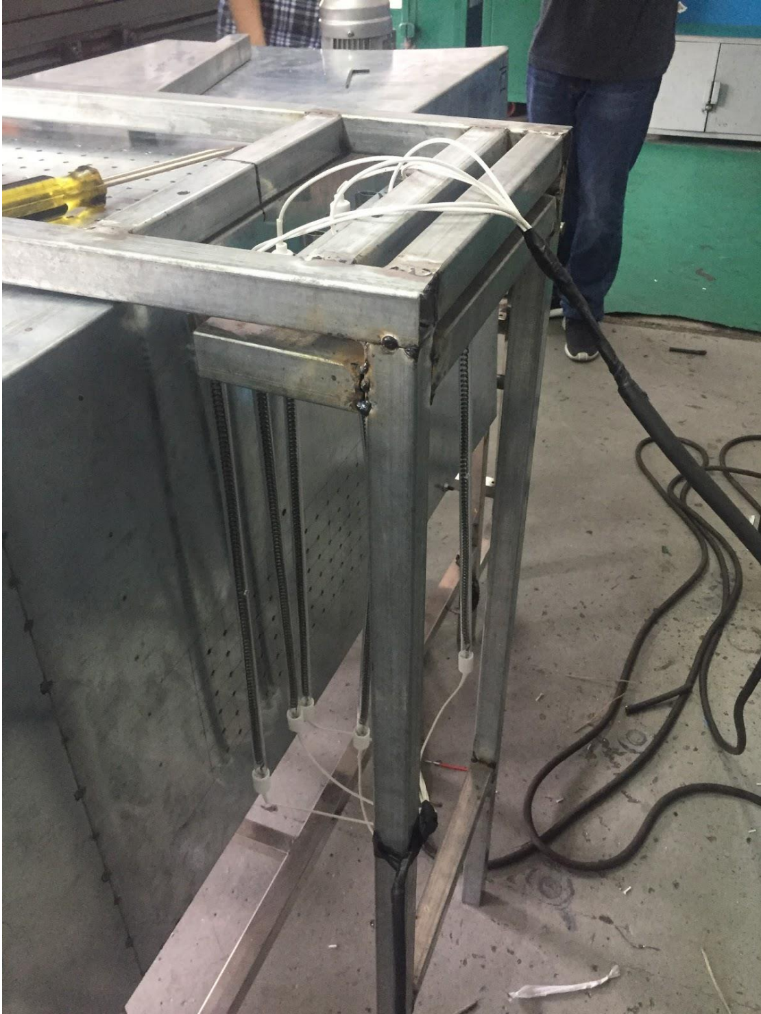
Figure 22: Ceramic Tubes Connected via Wires
