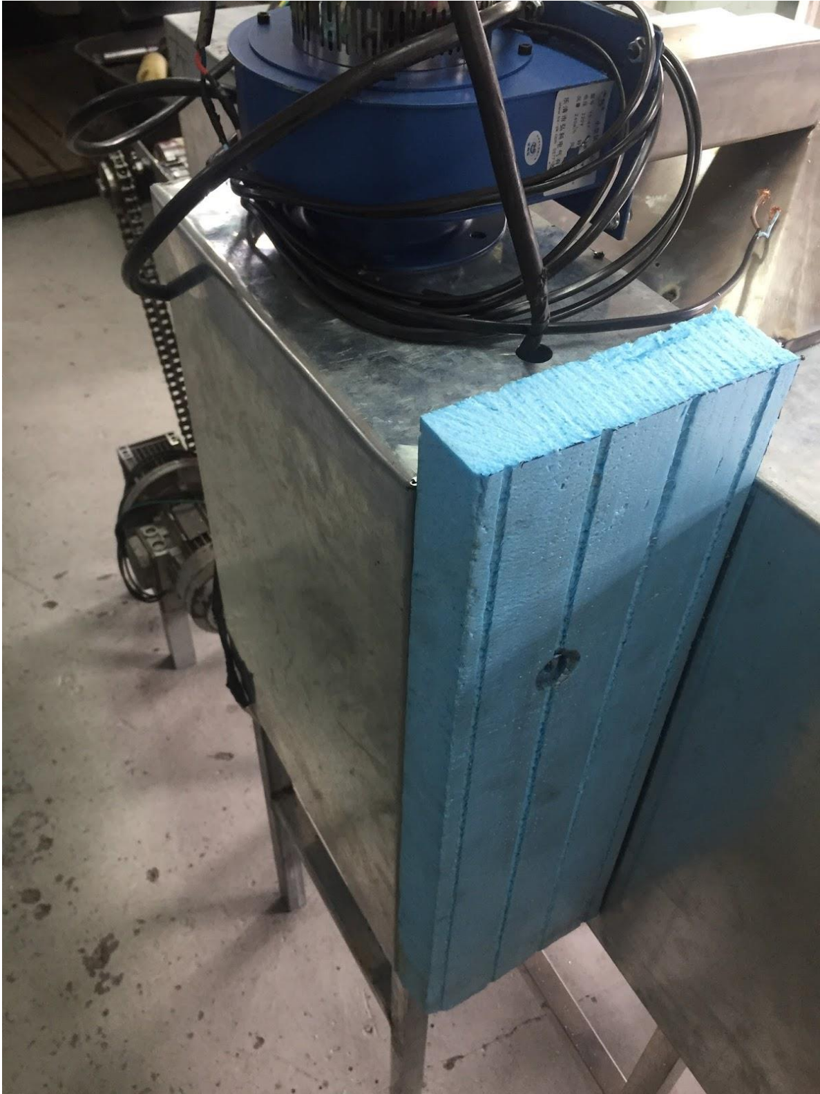
Figure 30: Insulation for the Heat Room
