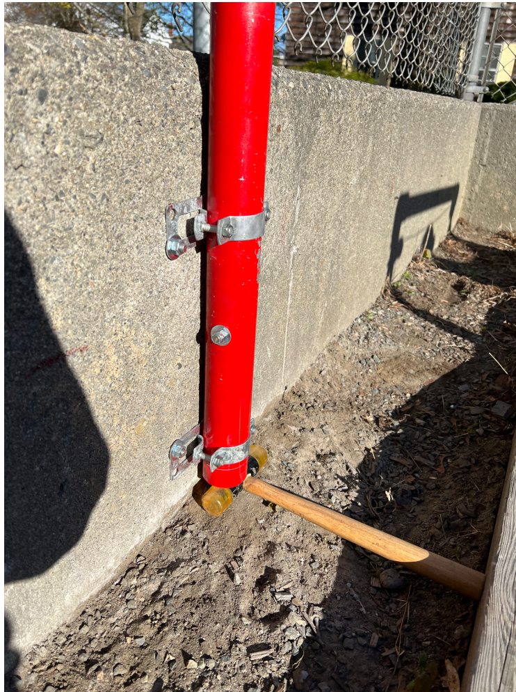
Figure 11: Red Post Elevated Off of the Ground During Installation
