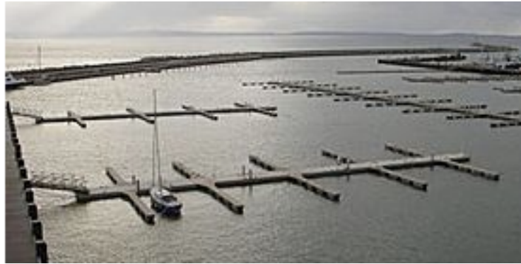
Figure 4-11: Pontoon mooring (Nautic Expo, 2011)
